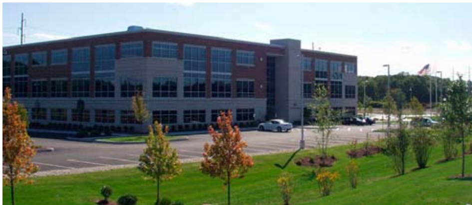
Metro East Office Park (Warwick, RI)
